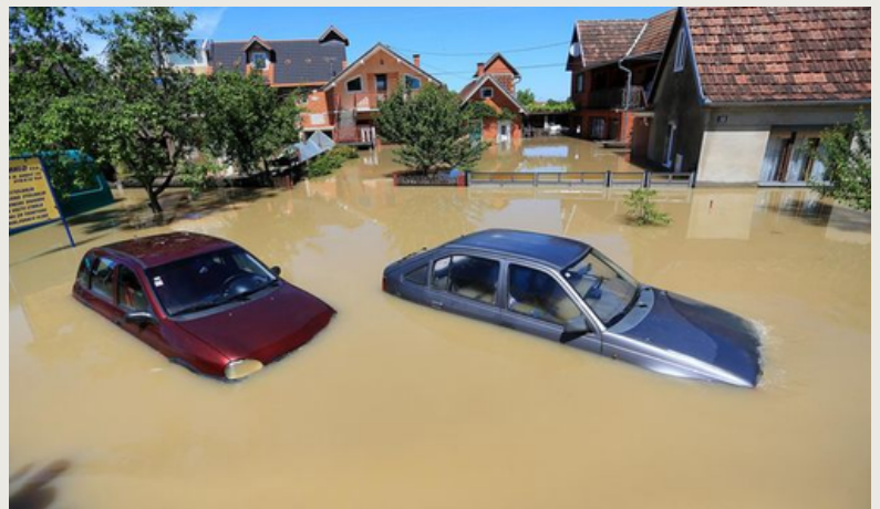
Figure 10: Damage caused by flooding
